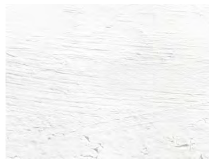
AF1 APPLIED FINISH TO MASONRY
