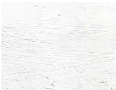
AF1 APPLIED FINISH TO MASONRY
